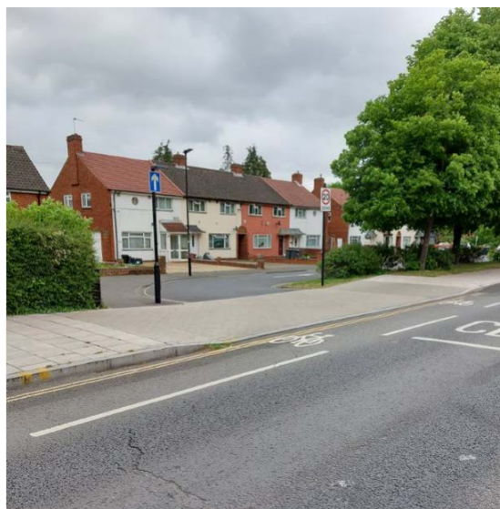
Image 1 – Example of a blended crossing on Bath Road, Hounslow
